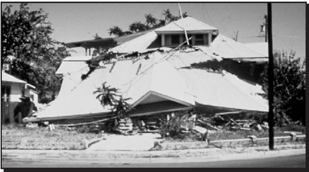
Additional damage from aftershocks
